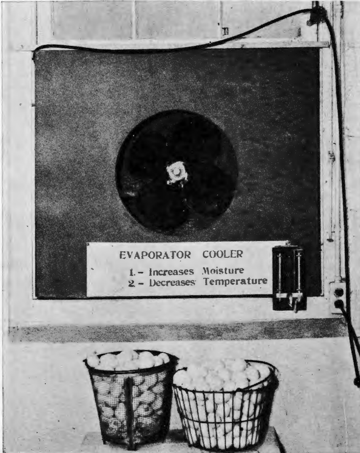
Figure 6. View of egg room cooler and humidifier from inside of egg room. Note two satisfactory egg gathering and holding baskets.
